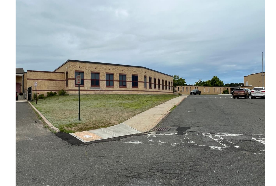
Figure 13: ADA/MAAB non-compliant crosswalk and curb ramps.
