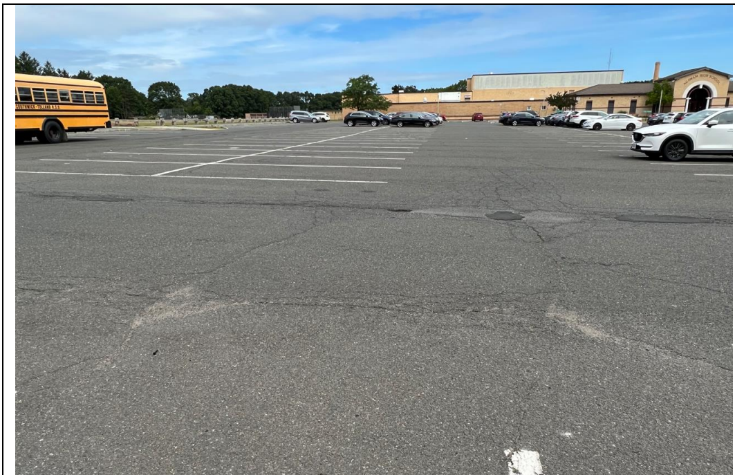
Figure 04: Longitudinal (Linear) and transverse cracking of bituminous paving in primary parking lot, with several patch areas also visible.
