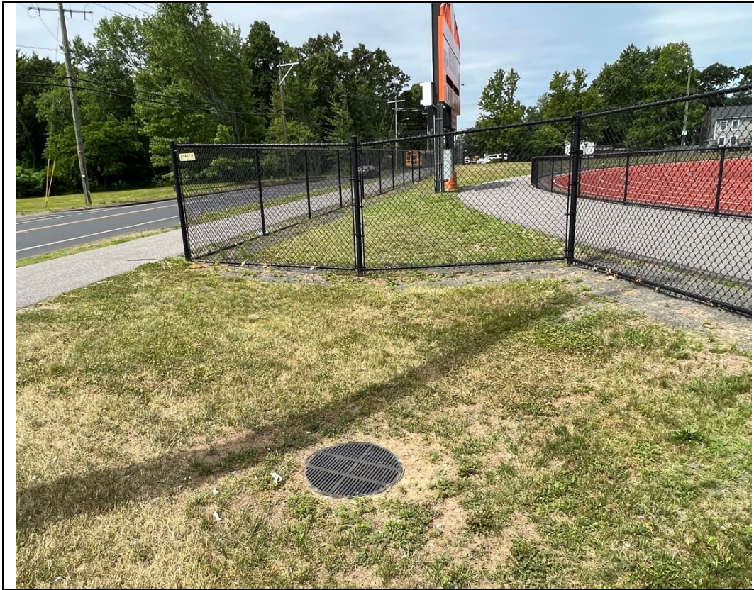
Figure 21: Typical condition of athletic facilities area drains
