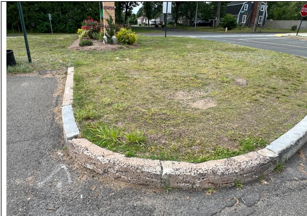
Figure 16: Typical condition of concrete curbing on the campus, in most cases disjointed and in poor condition.
