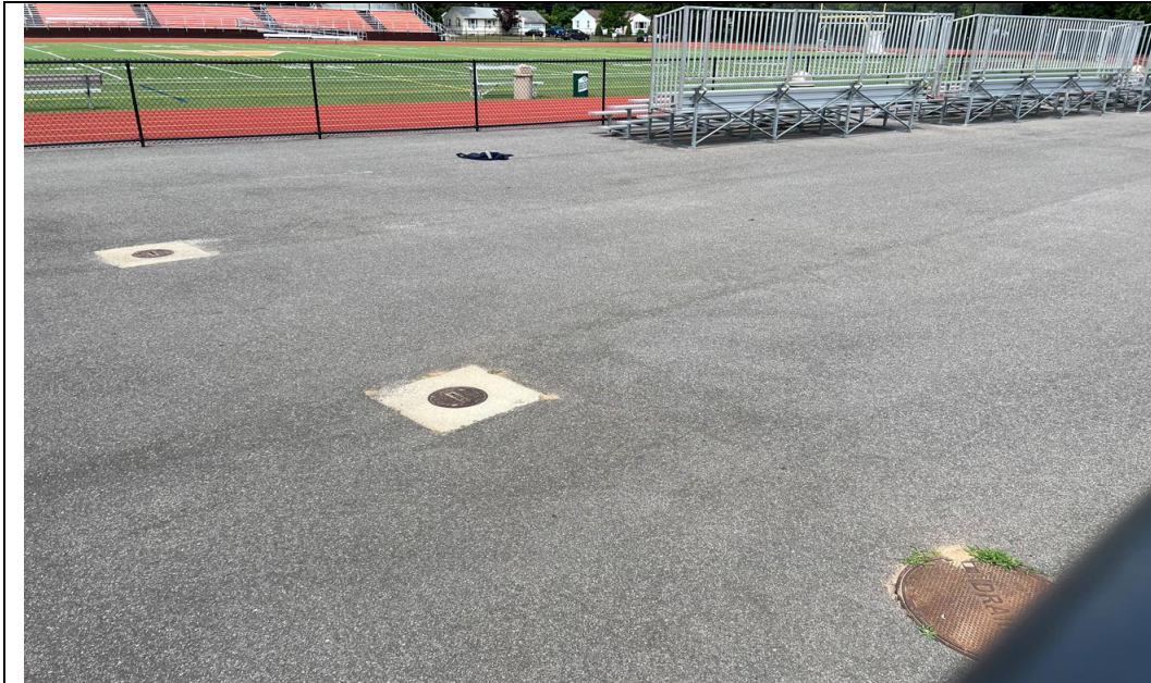
Figure 20: Track and field, with stormwater inspection ports and drain cover visible.
