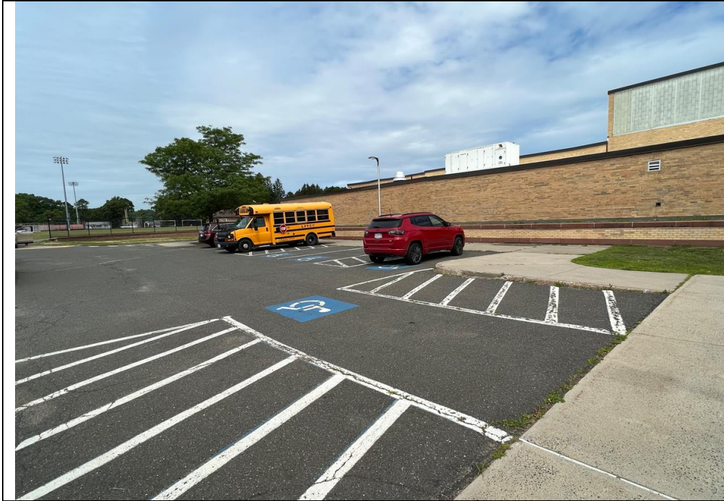
Figure 01: Main parking lot ADA parking area at the northwest corner of the main parking lot. All ADA areas should be checked for ADA compliant slopes and design.
