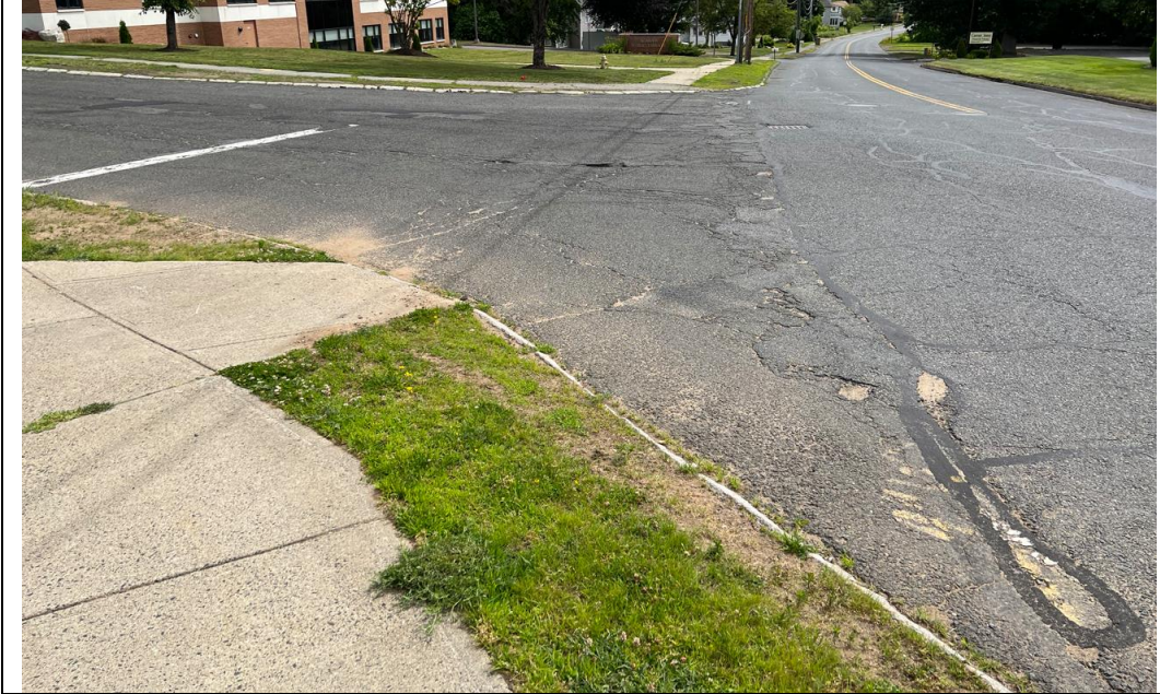
Figure 11: ADA ramp at the Cooper Street driveway entrance.
