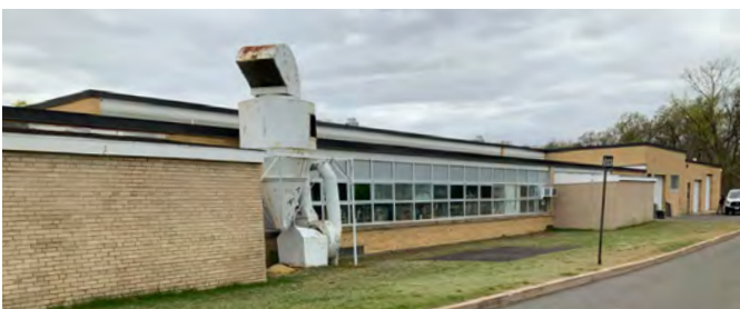
Lower Level East Facade
