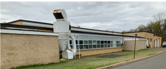
Lower Level East Facade
