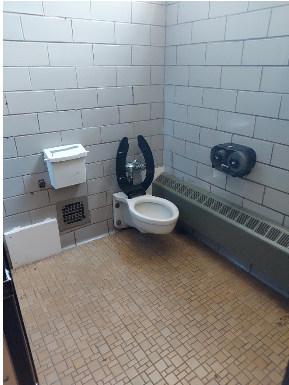
Lower Level Toilet Room
