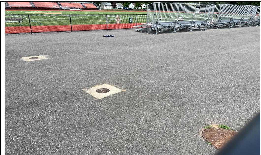
Figure 13: Track and field, with stormwater inspection ports and drain cover visible.
