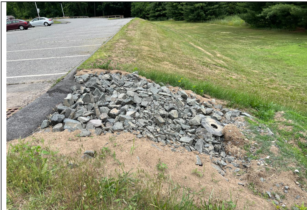
Figure 18: Rip rap at main DCB in the rear parking area, with debris and sediment noted. This area has clearly been a major erosion point and should be addressed with improved drainage infrastructure.
