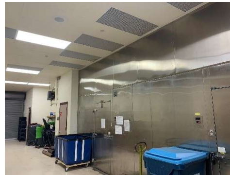
Kitchen walk-in coolers
