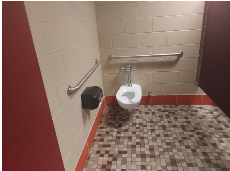
Locker Room Toilet Room
