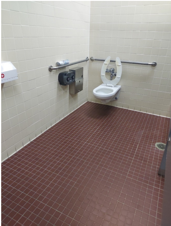
NW Toilet Room
