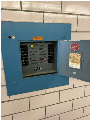
Recessed Hallway Panel
