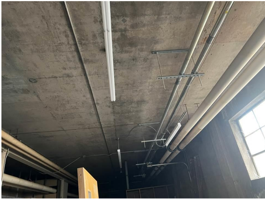
Second floor concrete slab supported on exterior concrete walls
