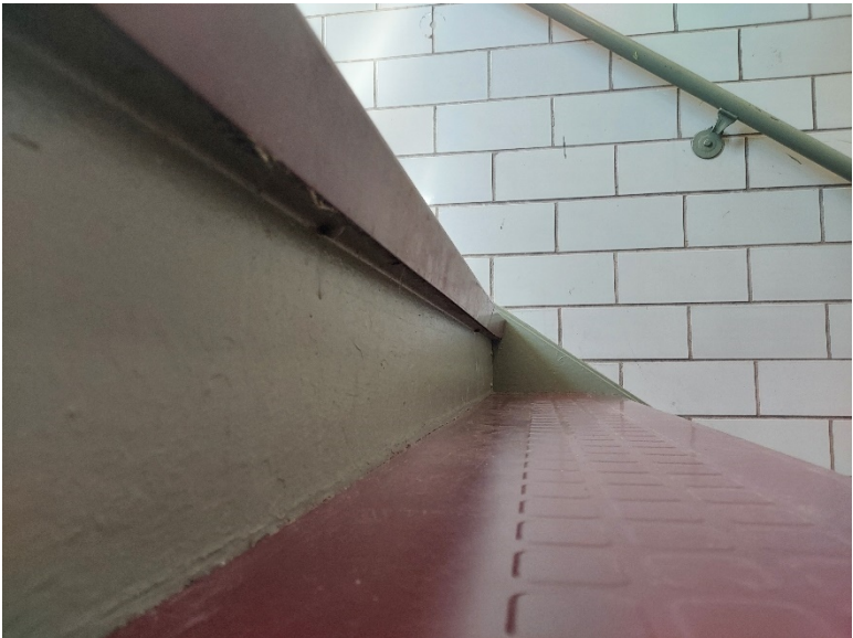
Lower Level Stair Nosings
