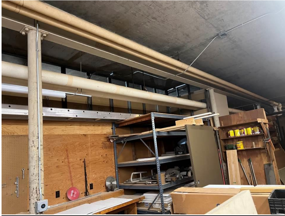
Typical second floor concrete slab supported on steel beams and columns
