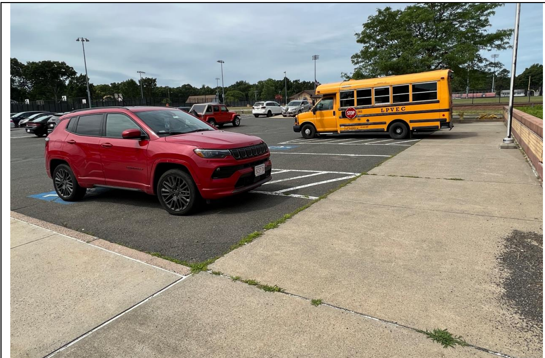
Figure 08: ADA parking spaces in the main parking lot.
