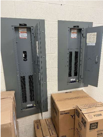
Loading Area Hallway
