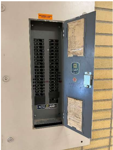
Recessed Hallway Panel
