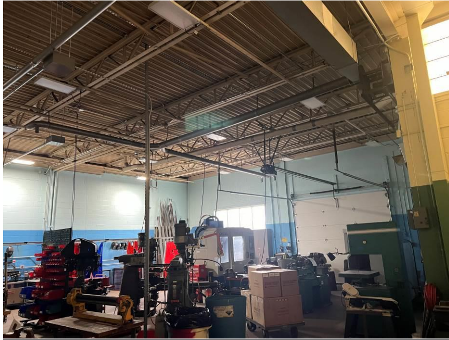
Typical roof framing at the shops
