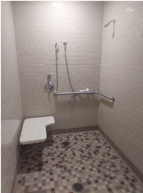
Boys Locker Room Shower
